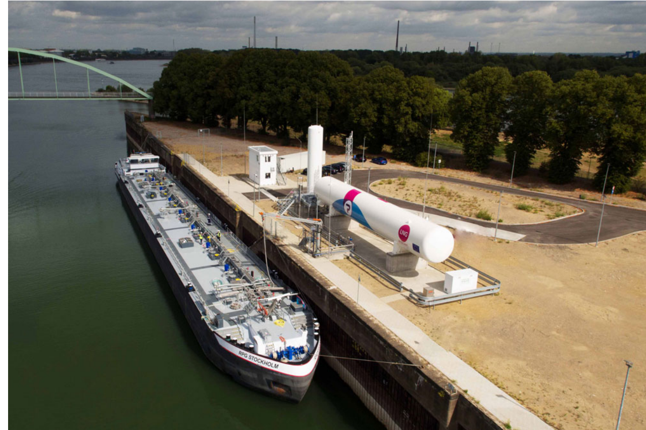
LNG tank in Germany's Port of Cologne / capacity up to 200 cubic metres
